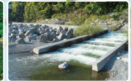
Fishway that was constructed in Toshima Dam
