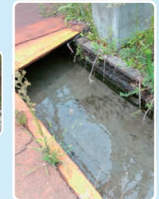
Monitoring of drainage at the Shimizu Plant of Nikkei Light Metal Co., Ltd.
